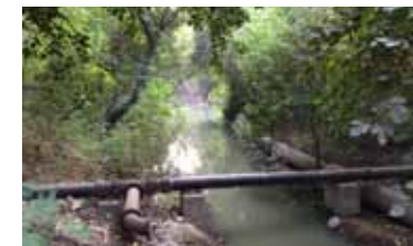
View of Existing Nullah at IIT
