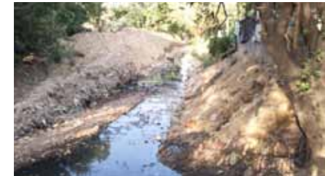
A. Existing Nullah Condition
